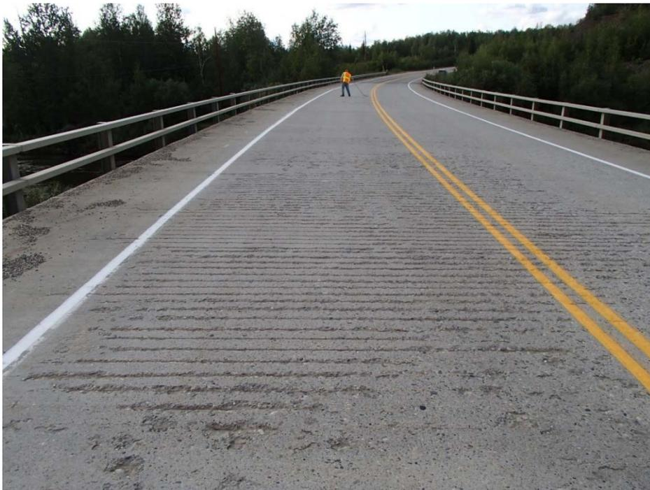
Figure 1: Damages on Chatanika River Bridge Deck
